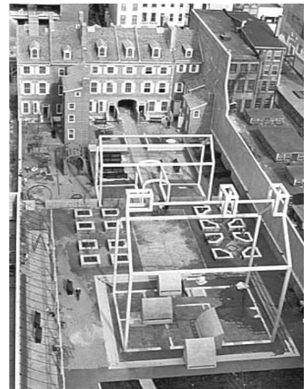
THE FRANKLIN COURT GHOST FRAME STRUCTURE DESIGNED BY ROBERT VENTURI IN PHILADELPHIA ALLOWS FOR INTERPRETATION WITH MINIMAL MAINTENANCE
