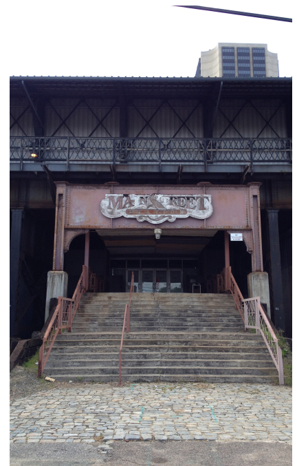
THE TERMINATION OF FRANKLIN STREET UNDER MAIN STREET STATION
