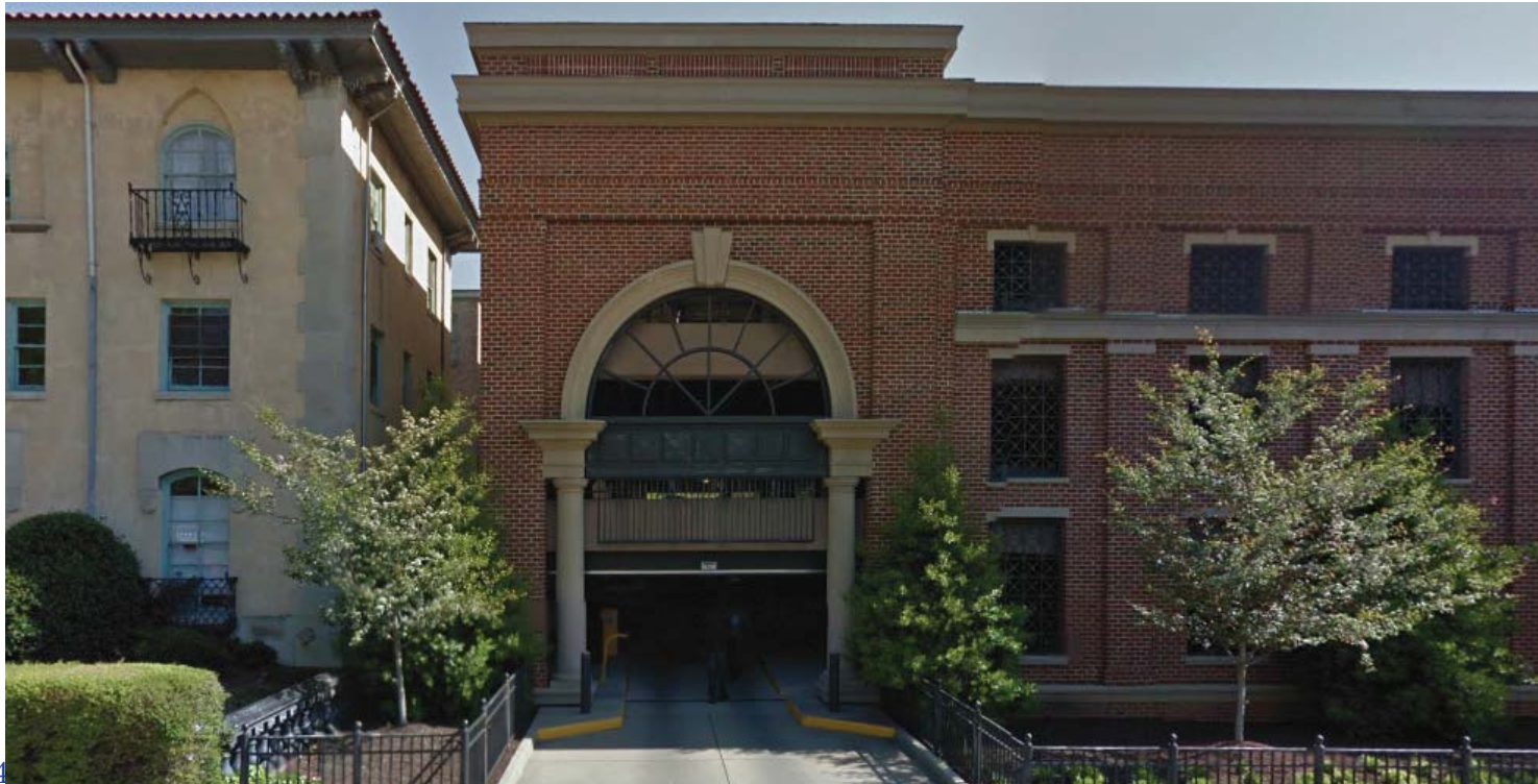
Photo 33: Appropriate parking structure on Franklin near Shafer stop is almost indistinguishable from its neighbors
