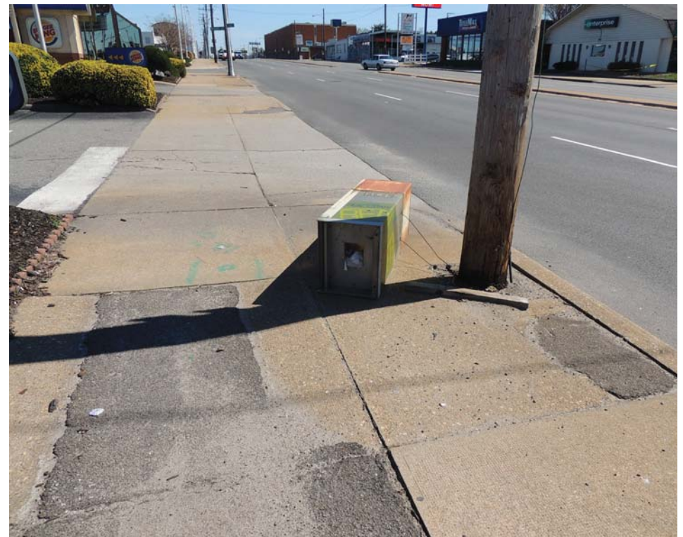
Photo 35: Low quality public space near Staples Mill W/ BRT
