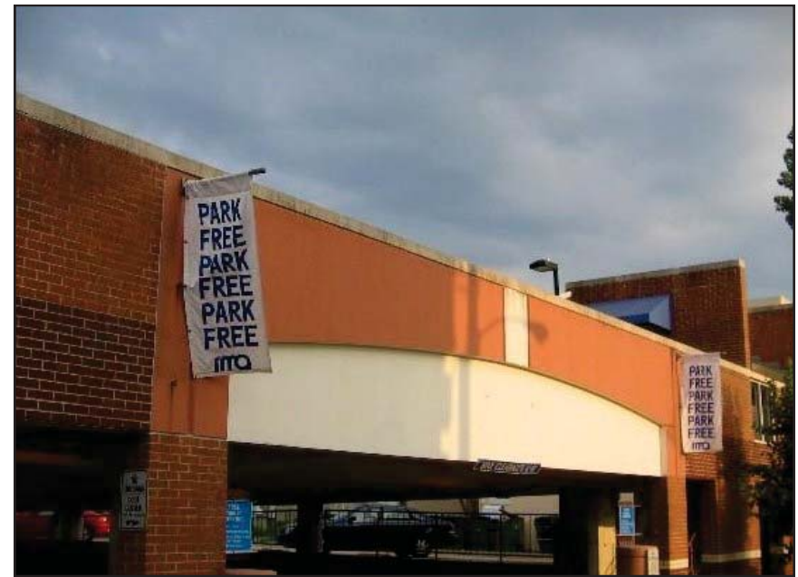
Image 33: A parking garage in Carytown helps ease the parking demand for the commercial district while reducing surface parking along the street frontage. A similar type of structure would be beneficial in the study area and the redevelopment of the 7 Eleven parcel should include a parking structure.
